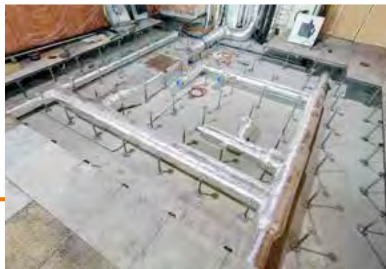
Primary air duct prepared for the installation of floor diffusers.
